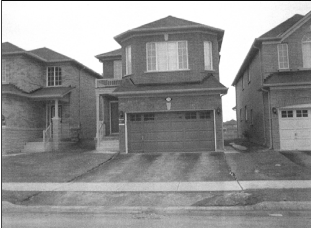
Photo 16: Consistent curb cuts at the street edge limit landscaping opportunities and the collective image of the street.
