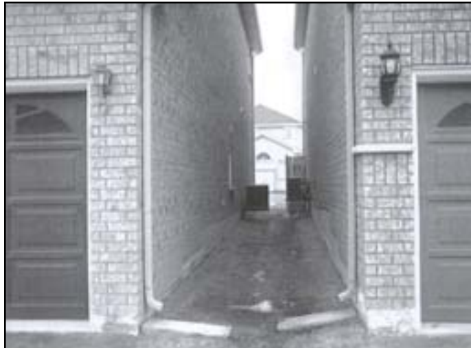
Photo 23: Encroachments into minimum sideyards prevents reasonable passage between houses and limits drainage
