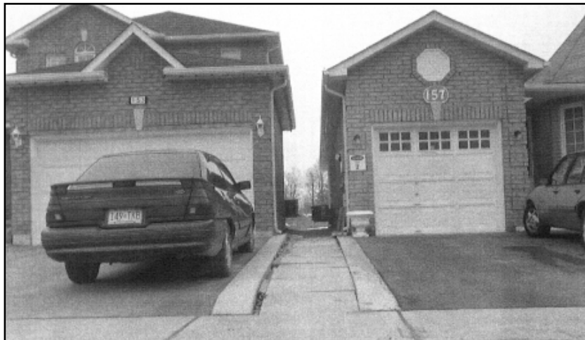
Photo 23: Encroachments into minimum sideyards prevents reasonable passage between houses and limits drainage
