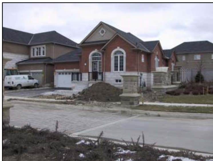
Photo 18: Current standards require community entrance features to be located on private property
