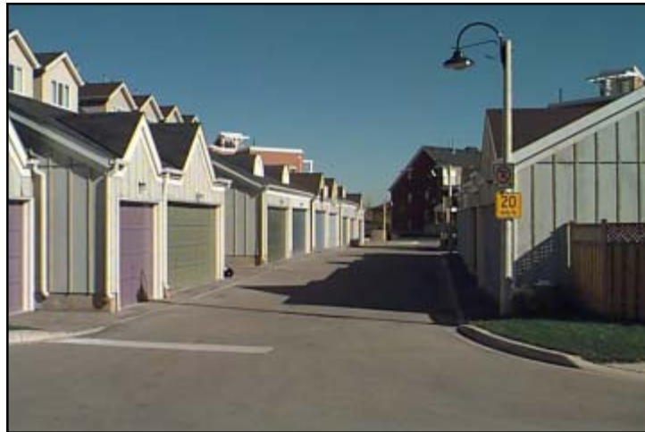
Photo 5: Access, safety and maintenance issues
