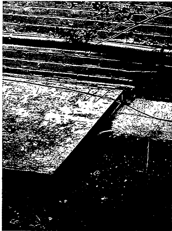
Hatch to basement, north elevation
