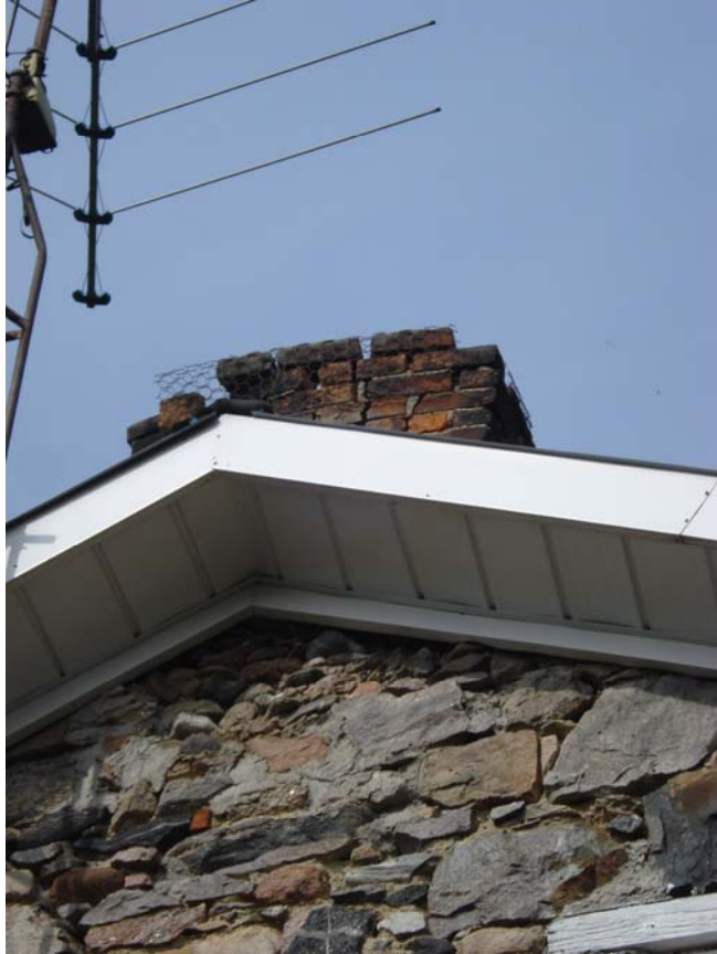
Figure 10 Spalling chimney with little remaining mortar, held together with chicken wire.
