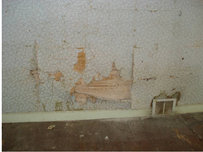
Figure 7 Exposed Lathe and Plaster on First Floor, Severely Water Damaged
