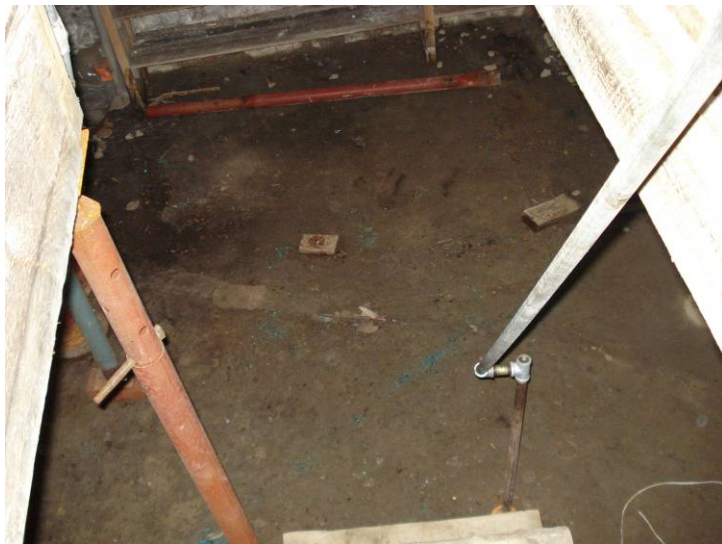
Figure 9 Large Crack in Basement Poured Concrete Floor, Recent Metal Support Post
