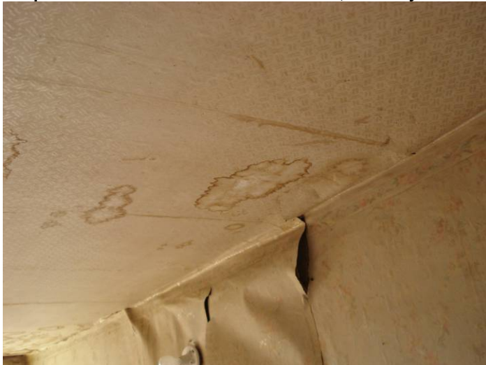
Figure 8 Upper Floor Water Damage, Through Attic and Down Walls
