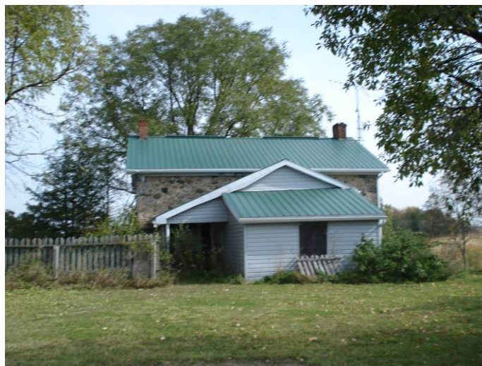
Figure 3 Rear Elevation of 12000 Highway 27
