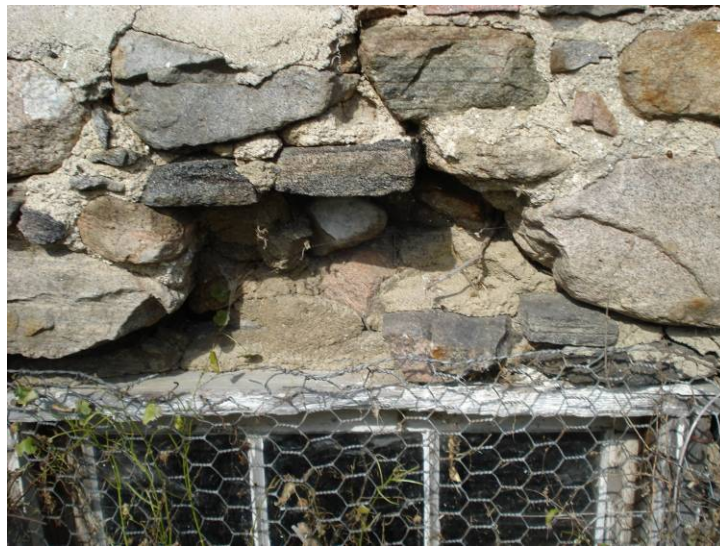
Figure 6 Secondary Stone Masonry Wall Exposed on the Southern Side Elevation
