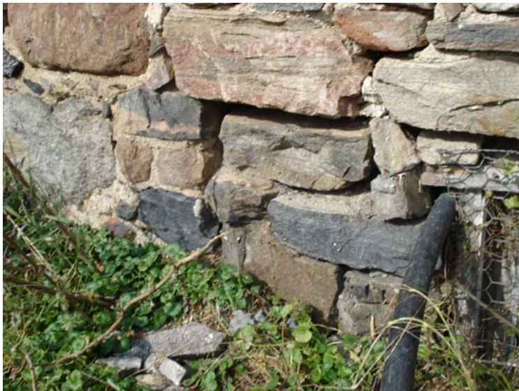
Figure 11 Failing stone masonry foundation.
