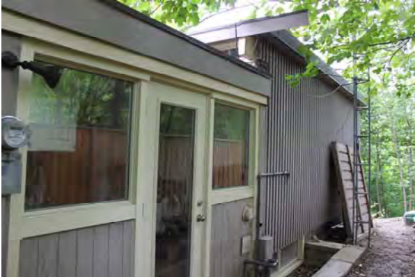
Fig. 20. North side yard and elevation view showing main portion of house. Barclay House, 82 Monsheen Drive, Woodbridge. Photo by Cultural Services, June 2011.
