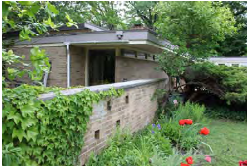
Fig. 18. South view at corner with east façade. Barclay House, 82 Monsheen Drive, Woodbridge. Photo by Cultural Services. June 2011.
