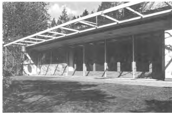
Fig. 10. B.C. Binning's house, West Vancouver, designed and built by owner. Image from Kalman.
