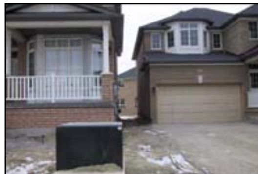
Photo 7: Encroachment into minimum standard side yards. Visibility of above-grade utilities.
