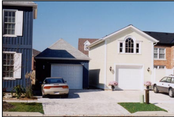
Photo 14: The garage and house can coexist through appropriate transitions of scale
