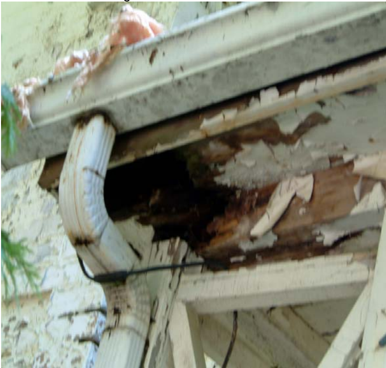
Damage to trimwork on west elevation
