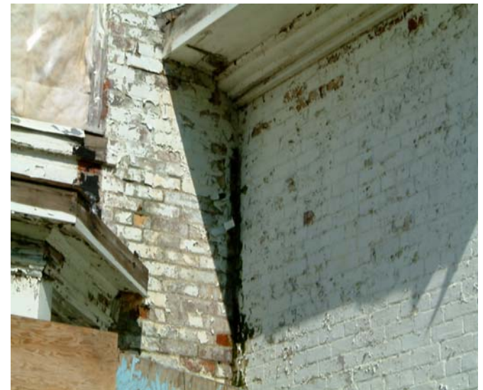
Wood deterioration by water/moisture at east elevation
