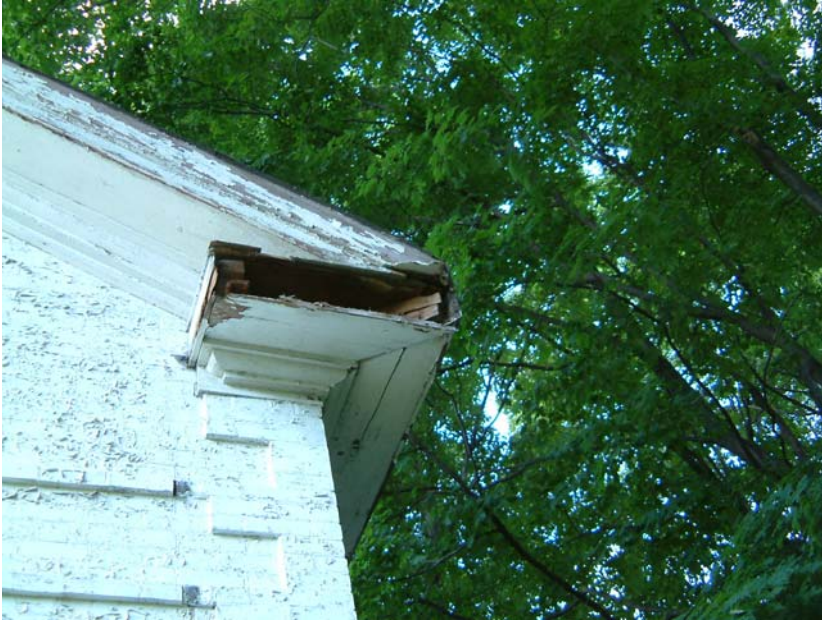
Damage to trimwork on west elevation
