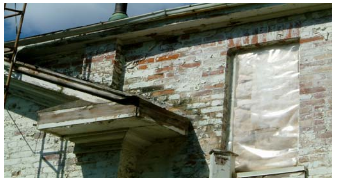
Wood deterioration by water/moisture at east elevation
