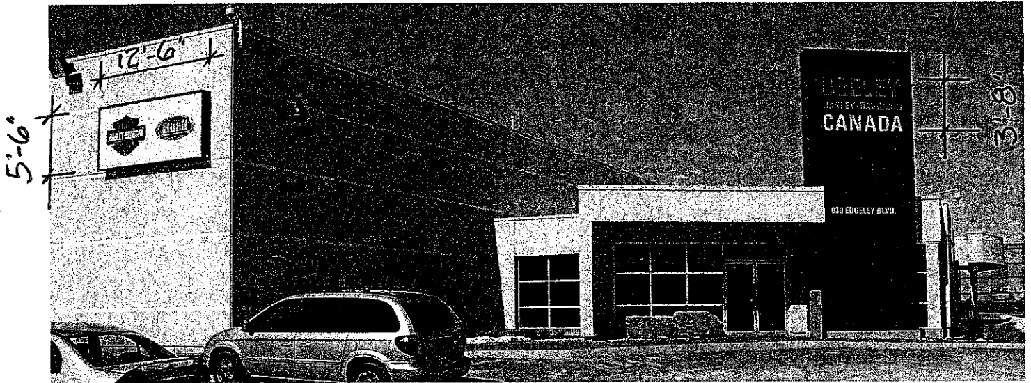
EXISTING SIGNAGE MARCH 7, 2006.
