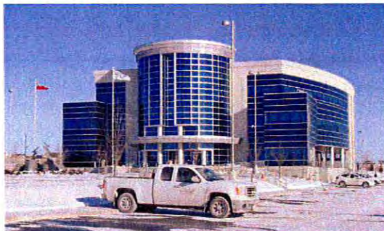
Figure 12: The Power Stream Building (LEED Standard) west of Highway 400
