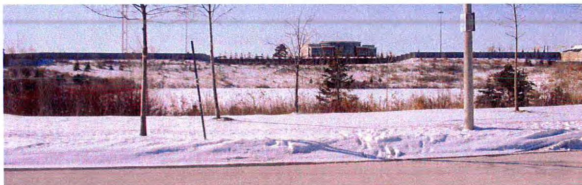
Figure 13: Large Storm Pond with Noise Fence and Highway 400 Beyond
