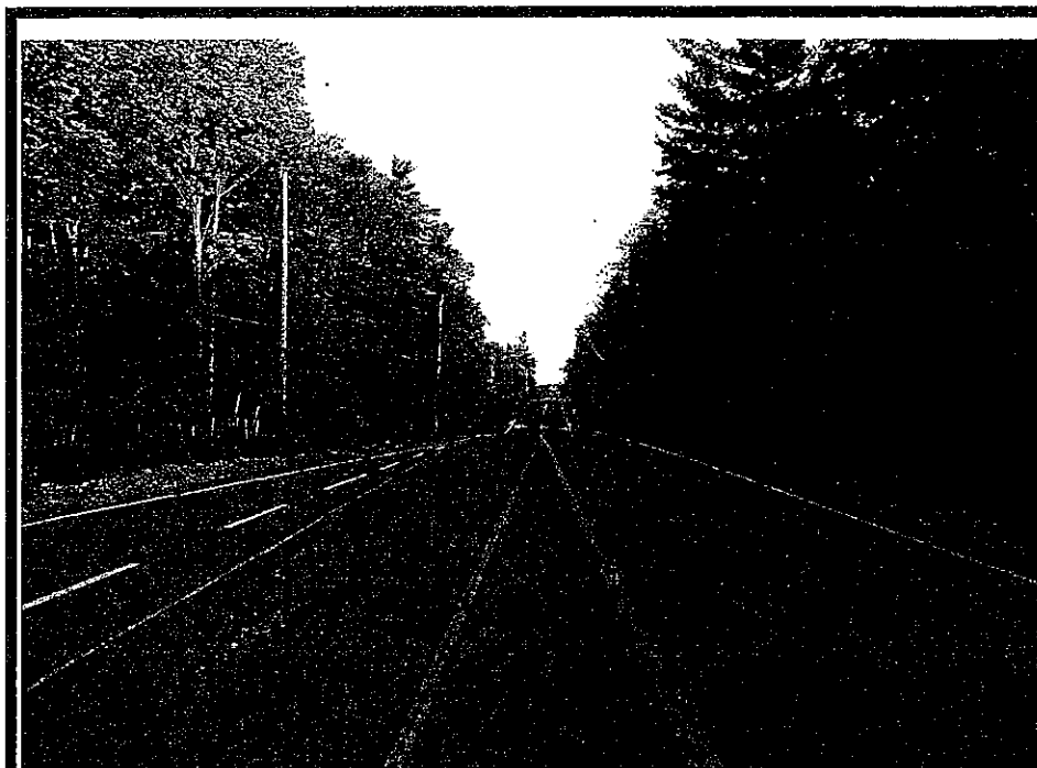
Pine Valley Drive looking south from Davos Drive adjacent to completed Block 39 urbanized residential neighbourhoods (May/2011)
