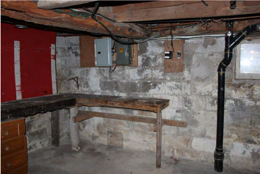
Fig. 13 to 16. Top to bottom: basement interior: block foundation wall, rough cut timber beam.
