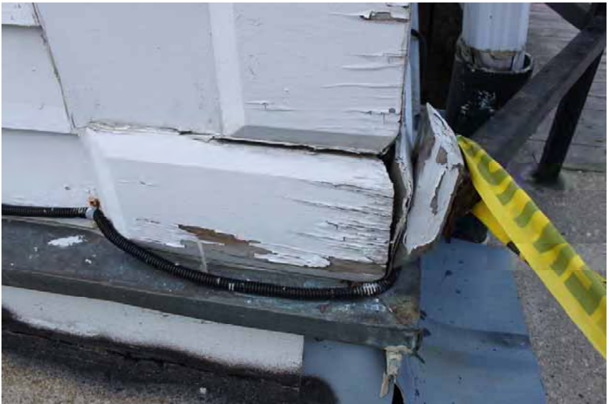
Fig. 5 Corner damage to exterior wood, 140 Brooke Street.
