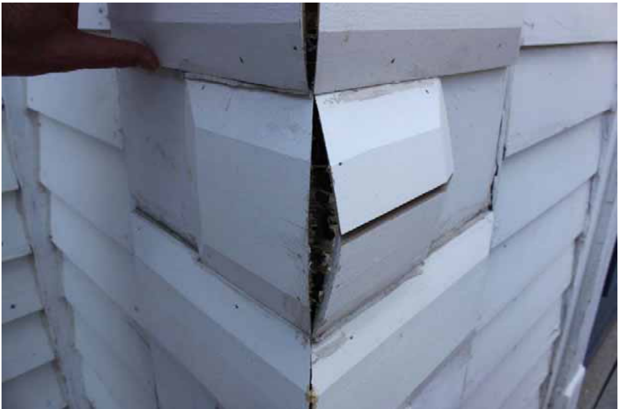
Fig. 6 Quoin water damage, bell tower, 140 Brooke Street.
