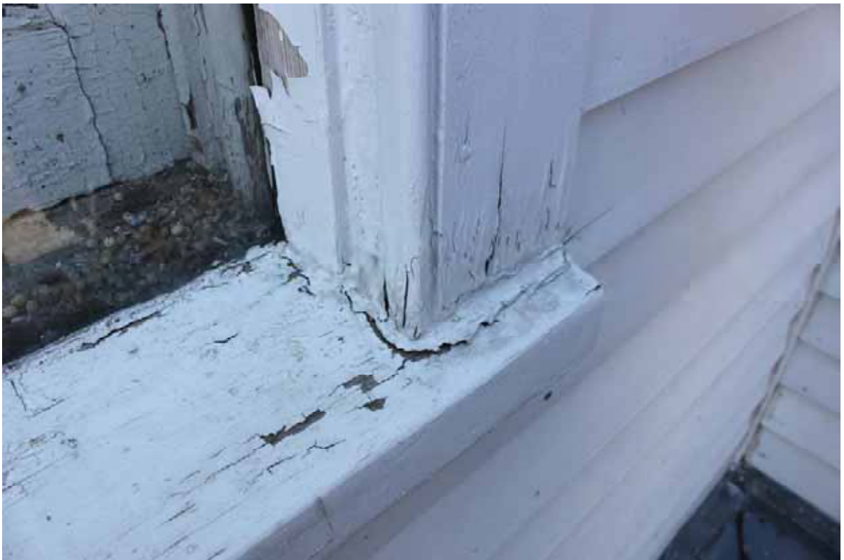
Fig. 7 Window frame water damage, 140 Brooke Street.
