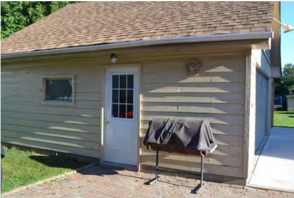
Fig. 3 July, 2012 – 942 Nashville Road, existing garage cladding. Photos by applicant.
