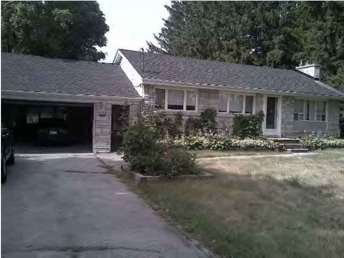
Fig. 2-4 July 9, 2012 Site Visit – 667 Nashville Road. Photos by applicant.
